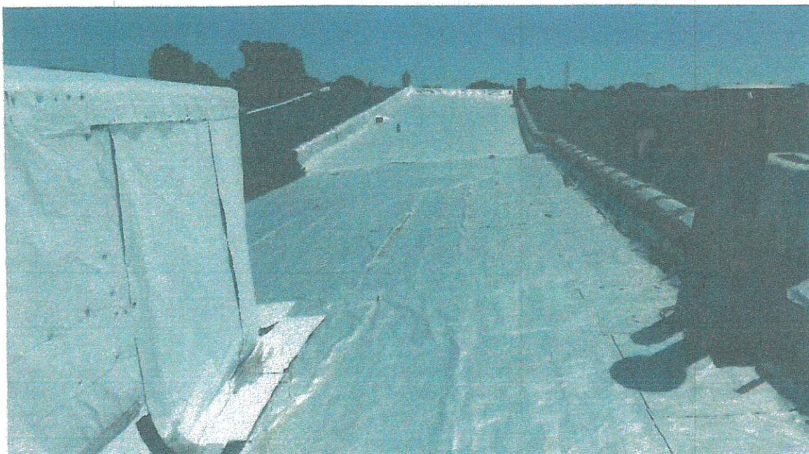
Photograph 5: Foil-faced membrane covering the roof and the access structure.
