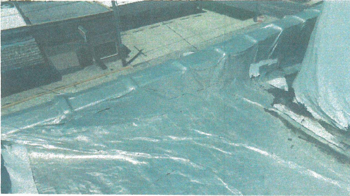
Photograph 9: No torn, displaced, or missing sections of the membrane along the west parapets.
