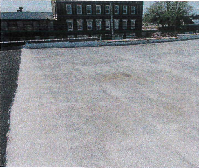
Photo 1: General view of the roof.
