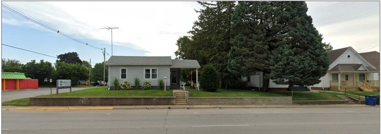
Figure 1. 721 North Main Street, Monmouth, IL as seen looking east from Main Street (28 Dec. 2020).
